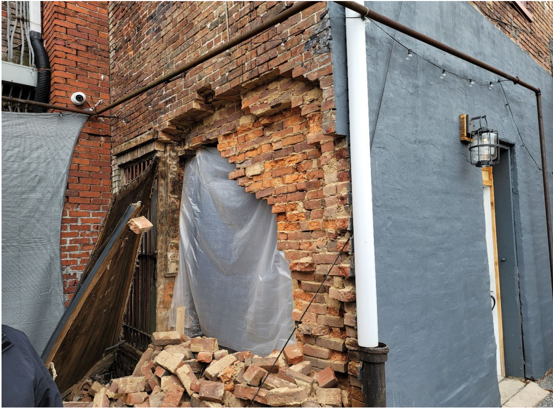
Photo 1. View of rear wall at collapse. Note window to the left of collapse.
