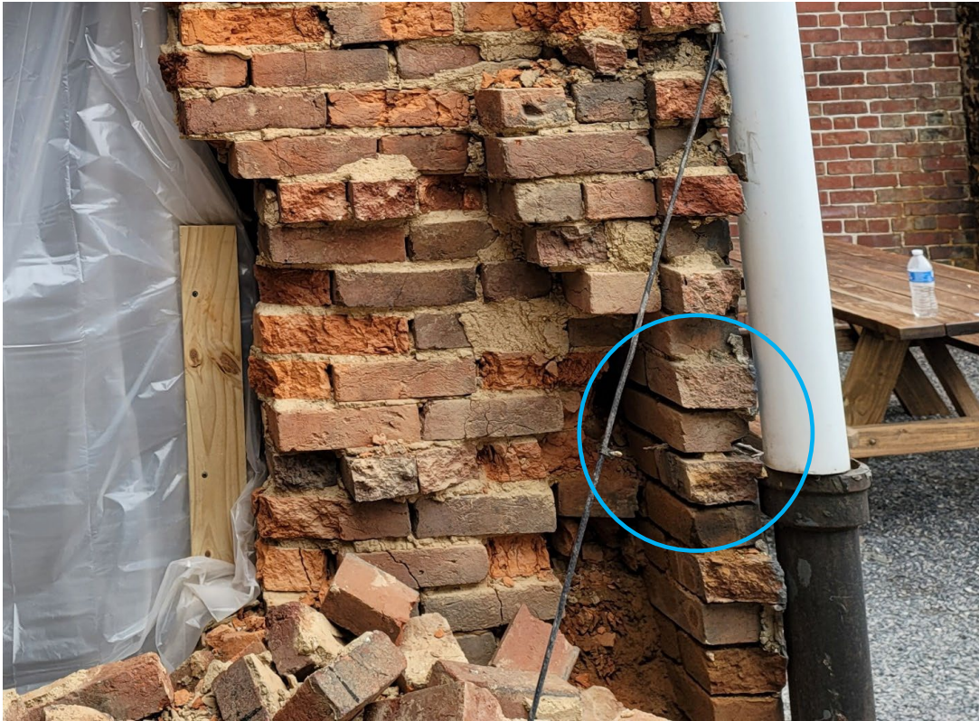
Photo 4. Detail of brick at corner. Interior brick fell apart at the touch. The arrow points to severely damaged brick. Note loss of mortar in exterior brick circled in blue.
