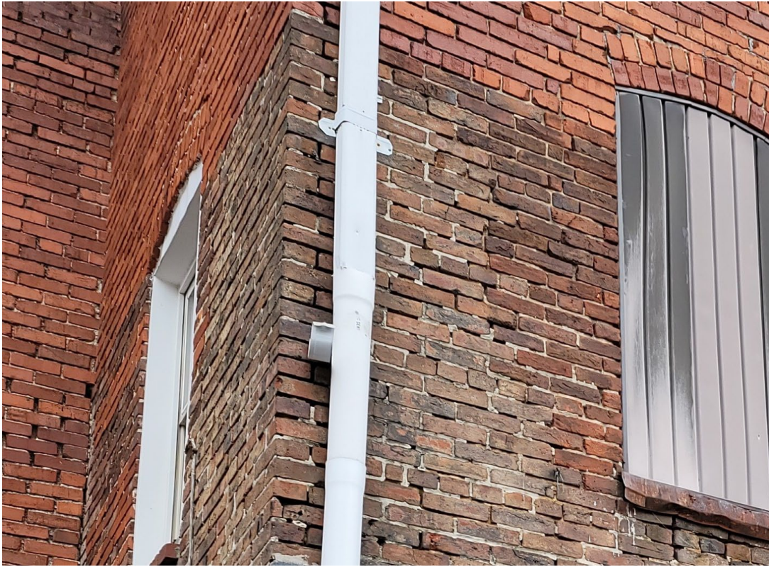
Photo 5. Note loss of mortar and staining at the corner of the wall near the downspout.
