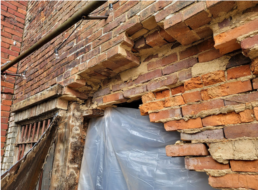
Photo 3. This view shows the side of the existing window. It is my understanding that there was a second window adjacent to it. Notice the delamination in the interior wythe.
