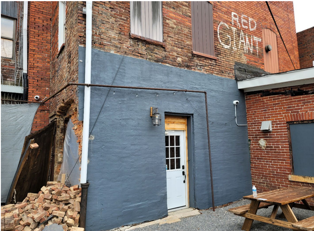
Photo 6. Rear of building adjacent to collapsed wall. Note wall was recently painted and appears to have been parged.
