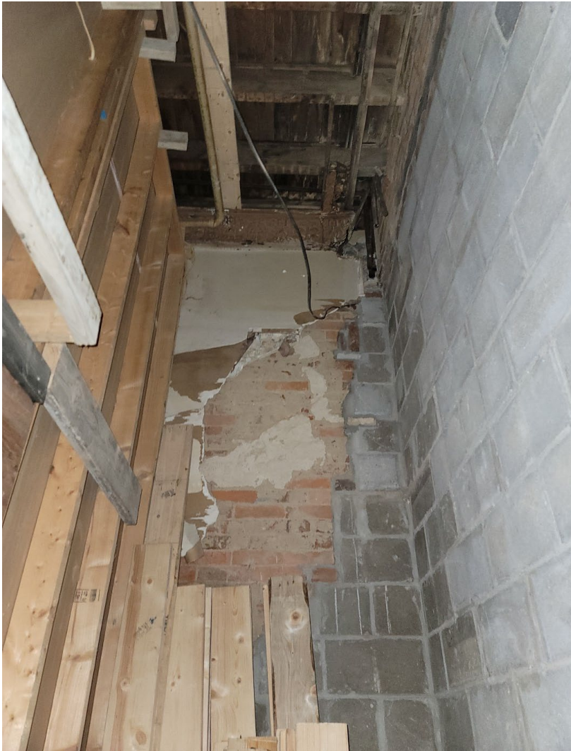
Photo 2. Completed work inside next to steps. The area of collapse was to the right. The corner on the right corresponds to the corner in the previous photograph.
