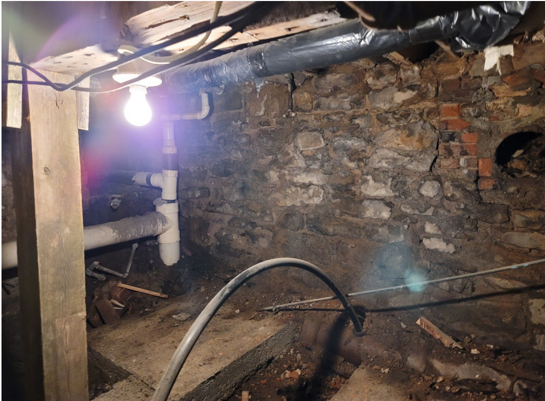
Photo 3. Repair work done in basement under collapsed wall included fixing damaged joists, supporting beam (essential for supporting upper levels while work was ongoing) and repointing the stone foundation.
